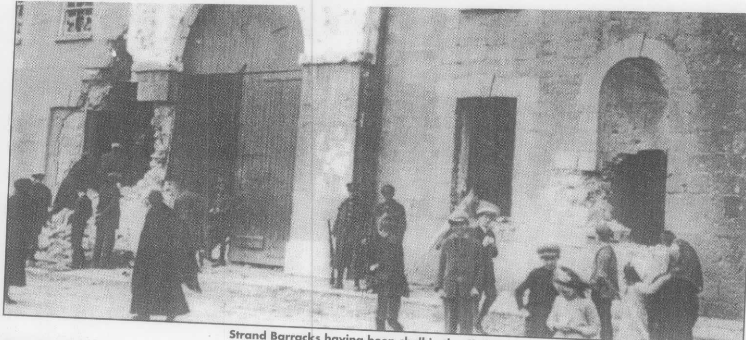
Strand Barracks having been shell in the Civil War
