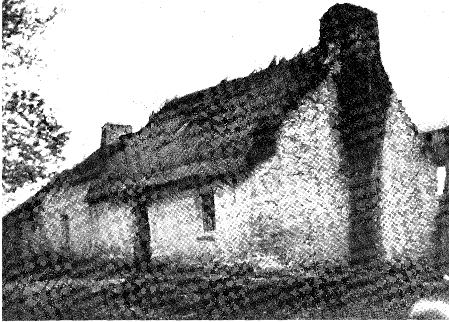
Cottage opposite Friar's Island, Killaloe
