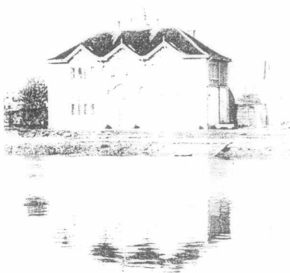
Watery grave: the submerged slipway
