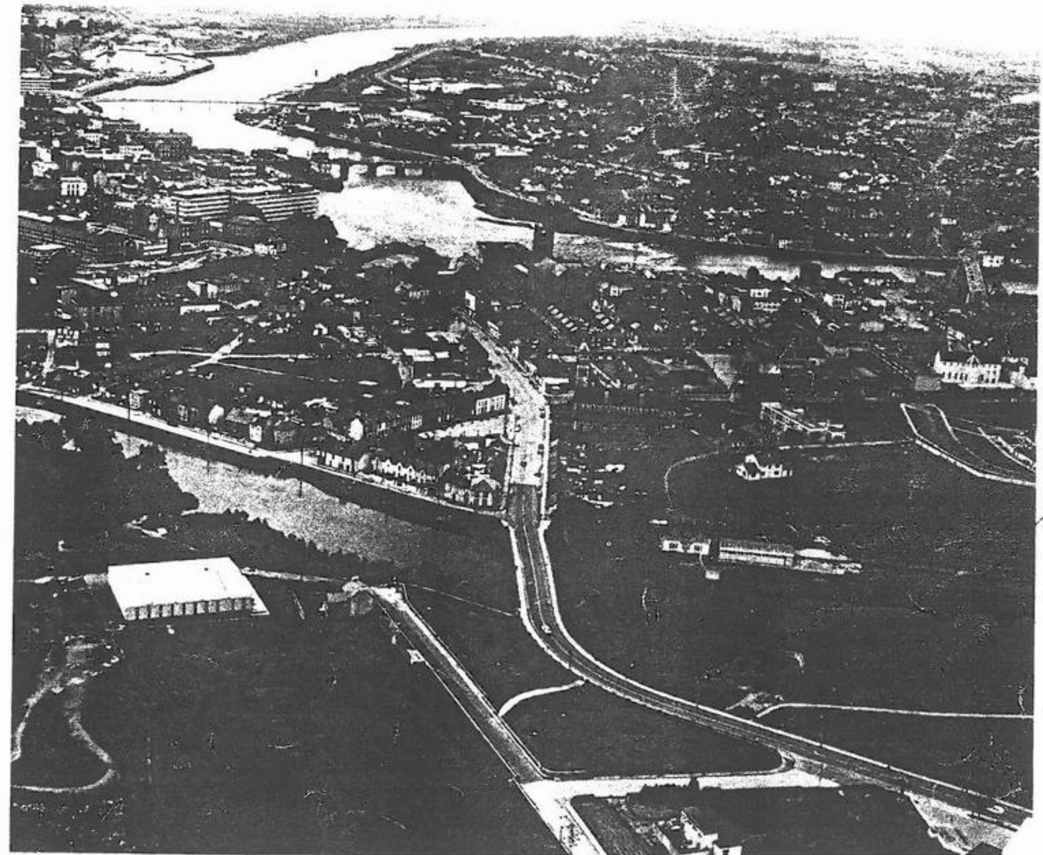
Below: Aerial view from Corbally over the Abbey and Shannon rivers.
