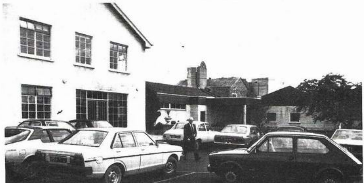
Shannon Meat Ltd. premises as seen from the water tanks.
