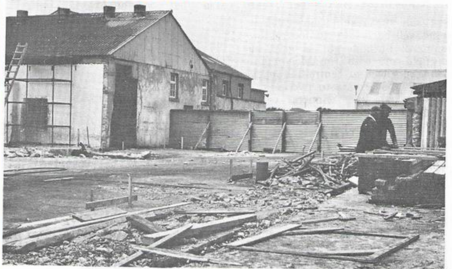
Preparing the site for the building of the new abbatoir - 1970.
