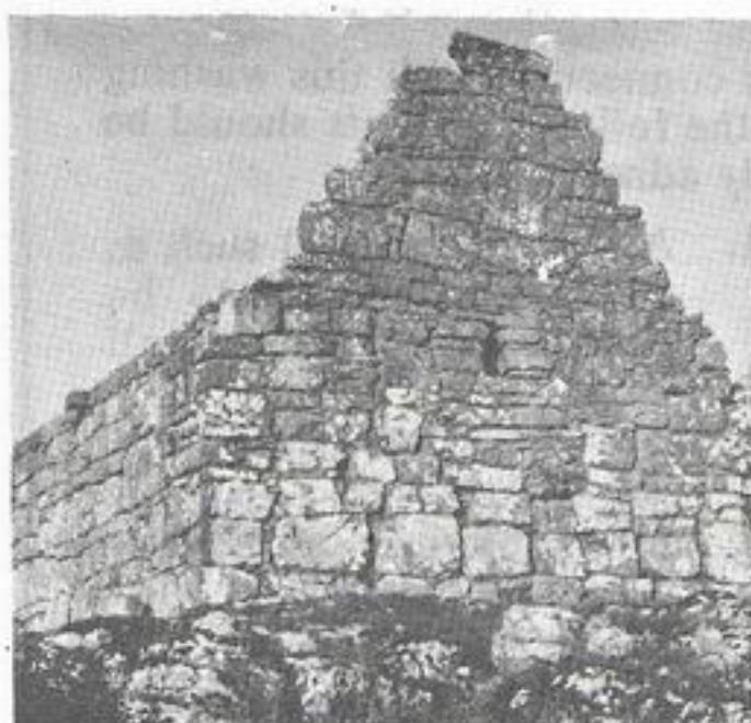
KILLULTA: East gable and south wall showing rock outcrop on which oratory was built.
