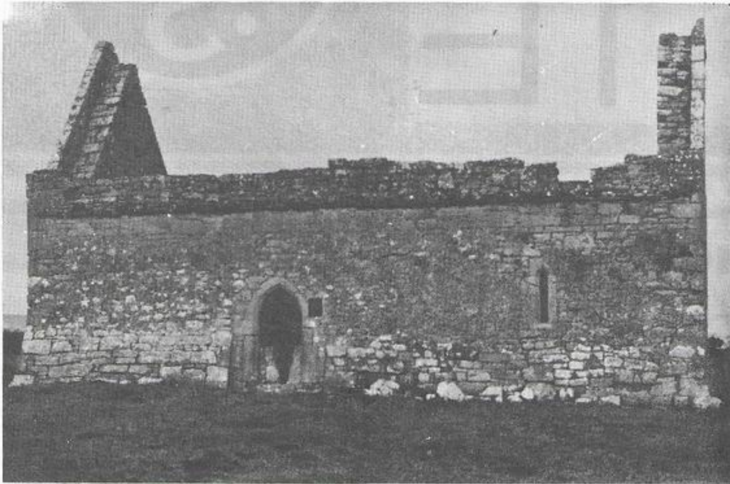
KILLEEN: General View of Church from the south, showing pointed doorway, ogival headed window, gutter outlets along top of wall, roof seating in gables and battered wall base. All Photos by Author.
