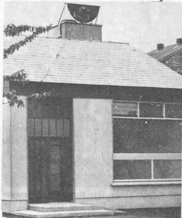
An external view of the new Display Area.
