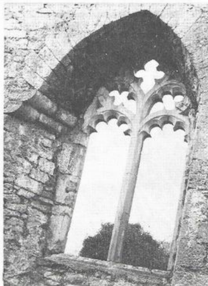
Askeaton Friary: Window in North wall of Choir of Church with cusped "flowing" tracery.
