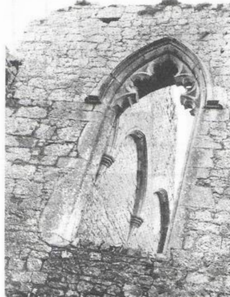
Askeaton Castle: The Banqueting Hall; Traceried Window in last wall with pointed hood moulding and view of blind arcading inside.
