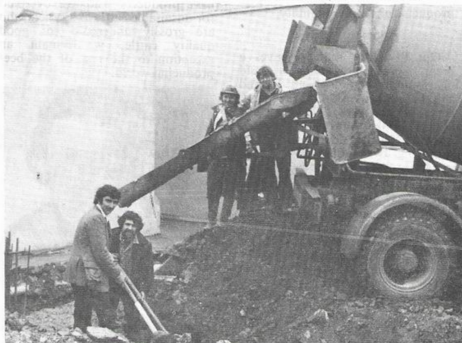
Busy building the Can Goods Store are Frank Costelloe, K. Carmody, B. Ryan and T. O'Leary.
