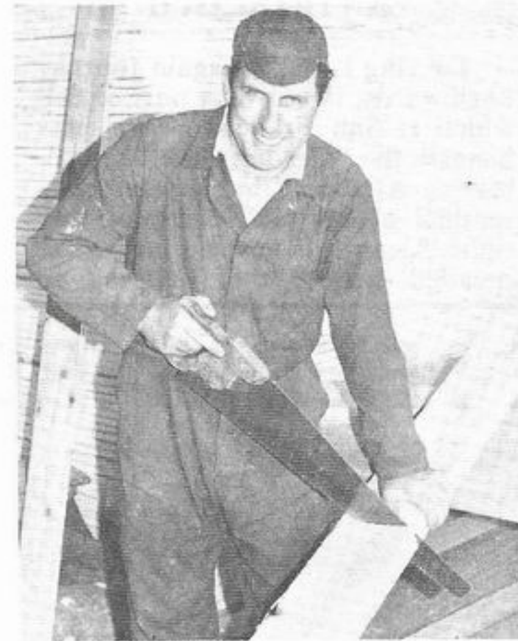
Michael Morrissey busy in the Civil Workshop.
