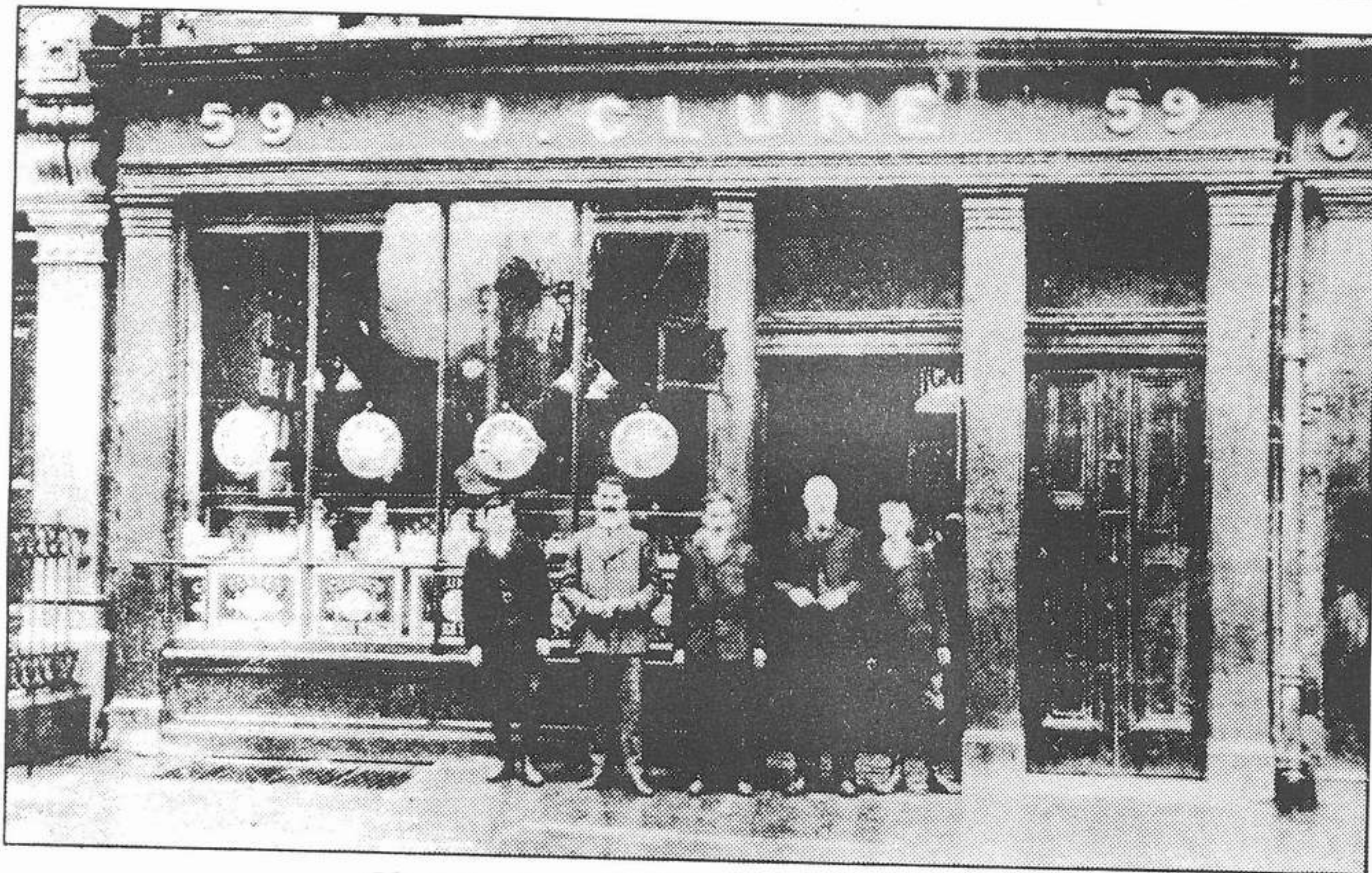
Clune's shop, William Street, c. 1910.
