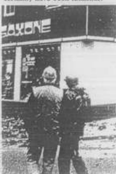
Workers prepare to demolish the building.
