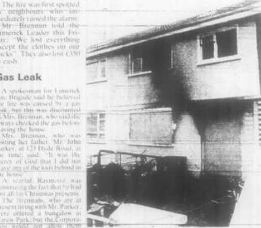
Aftermath of the fire.
