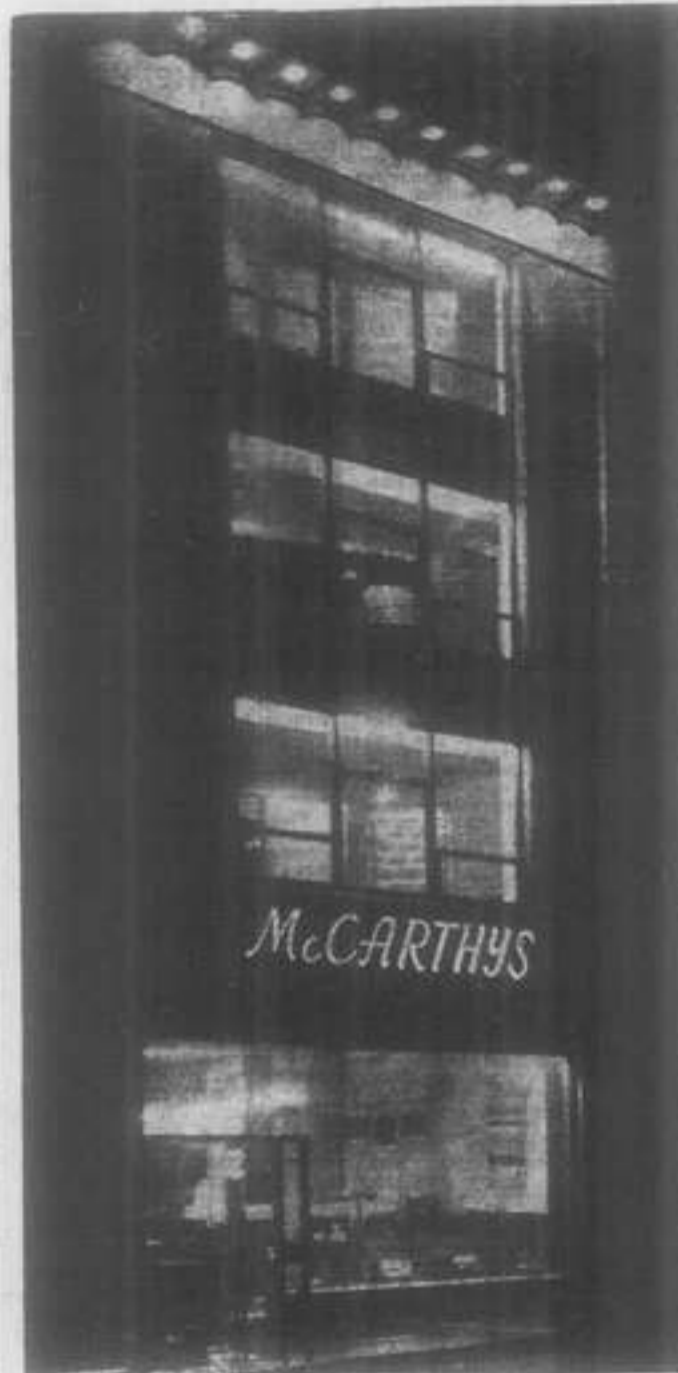
An impressive view of McCARTHY'S New Frontage.
