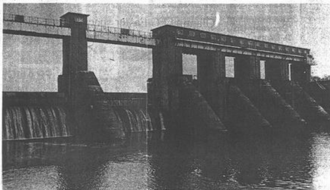
Parteen-a-lax weir lets down ten tonnes of water a second. The other 168 tonnes make electricity.
