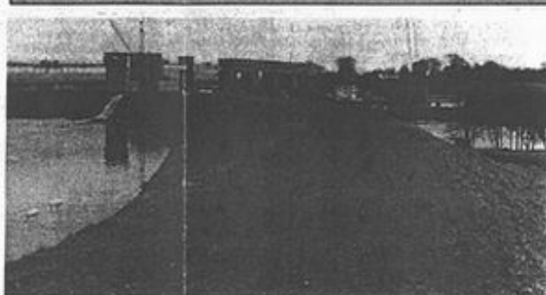
The high and the low of it. The headrace (left) takes most of the Shannon flow, while the old river (right) receives ten tonnes of water each second to keep the ecology going. The difference in height is some 15 metres at that stage.
