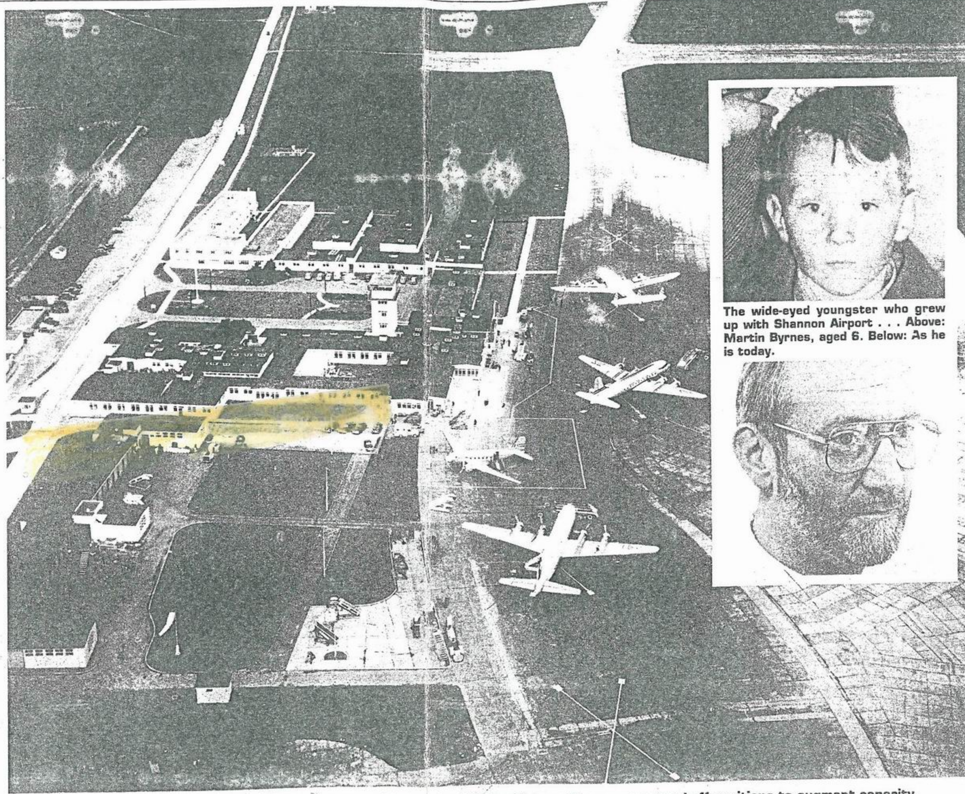
Some of the seven inner airstands are occupied in this late 'fifties picture. There were stand-off positions to augment capacity.
