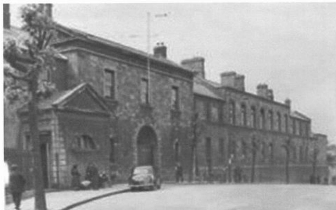
South Dublin Union Workhouse
