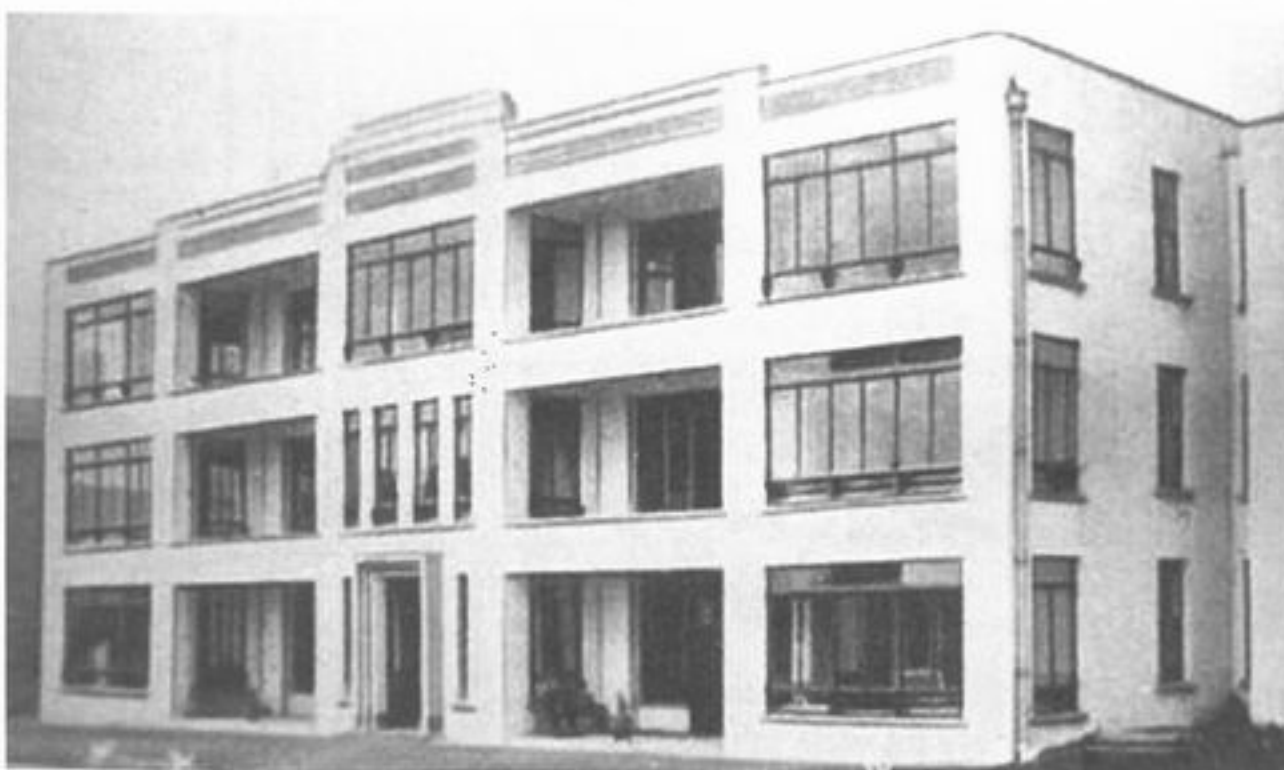
New tuberculosis hospital after completion from Brendan Connellan Light on the past, Story of St Mary's Limerick 1838-1938 (Limerick, 1938), p.60
