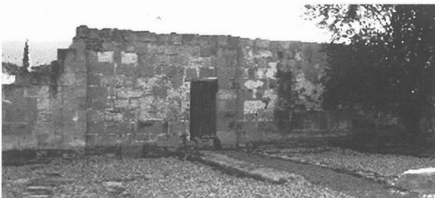
Remaining walls of Cascades Female Factory
