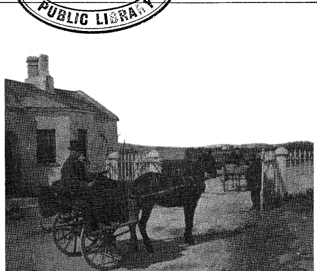
The toll gates at Athlunkard Bridge.
