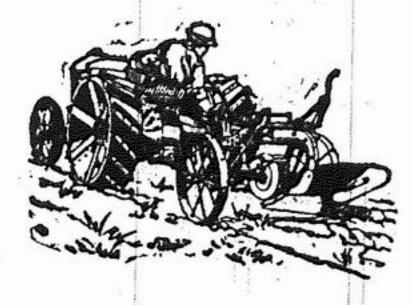
FORDSON TRACTOR delivered to purchaser. 22 horse power, 3 speed and reverse, Weight 28 owts, Length 8ft Sin, Width 5ft 2in. Height 4ft 4in Price (at Works, Cork), £235. Extra for puly attachment £10 10e 0d. Read bands for wheels £6 0e 6d.
