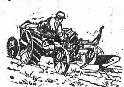
Fondson Tractor delivered to purchaser. 22 horse power, 3 speed and reverse, Weight 23 owts, Length 8ft 6in, Width 5ft 210, Height 4ft 4in Price (at Worke, Cork), £235. Extra for puly attachment £12 10a 0d.
