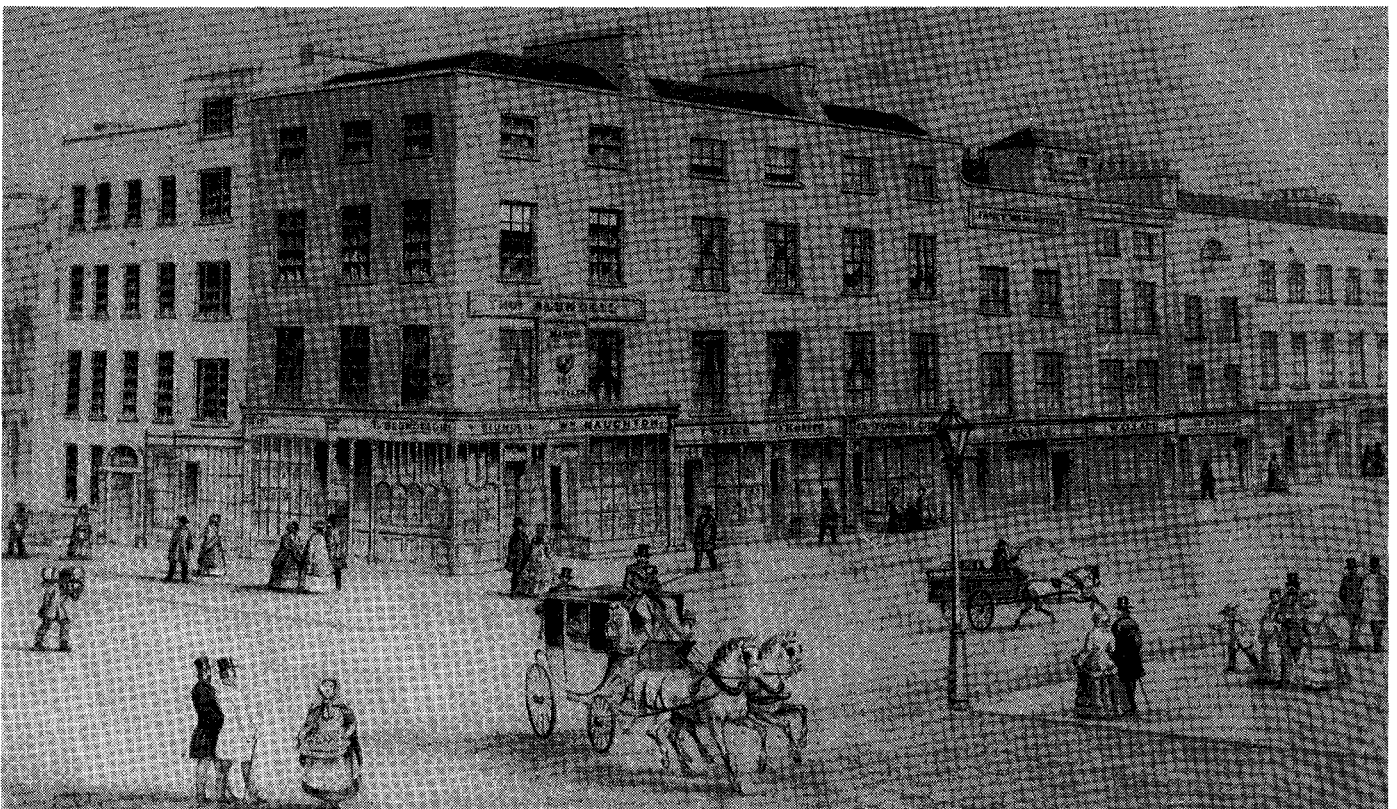
A mid-nineteenth century view of Newtown Pery.
