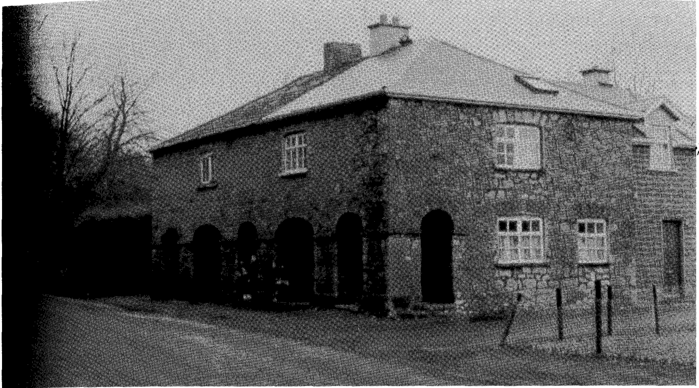
Ahane School in February, 1992.
