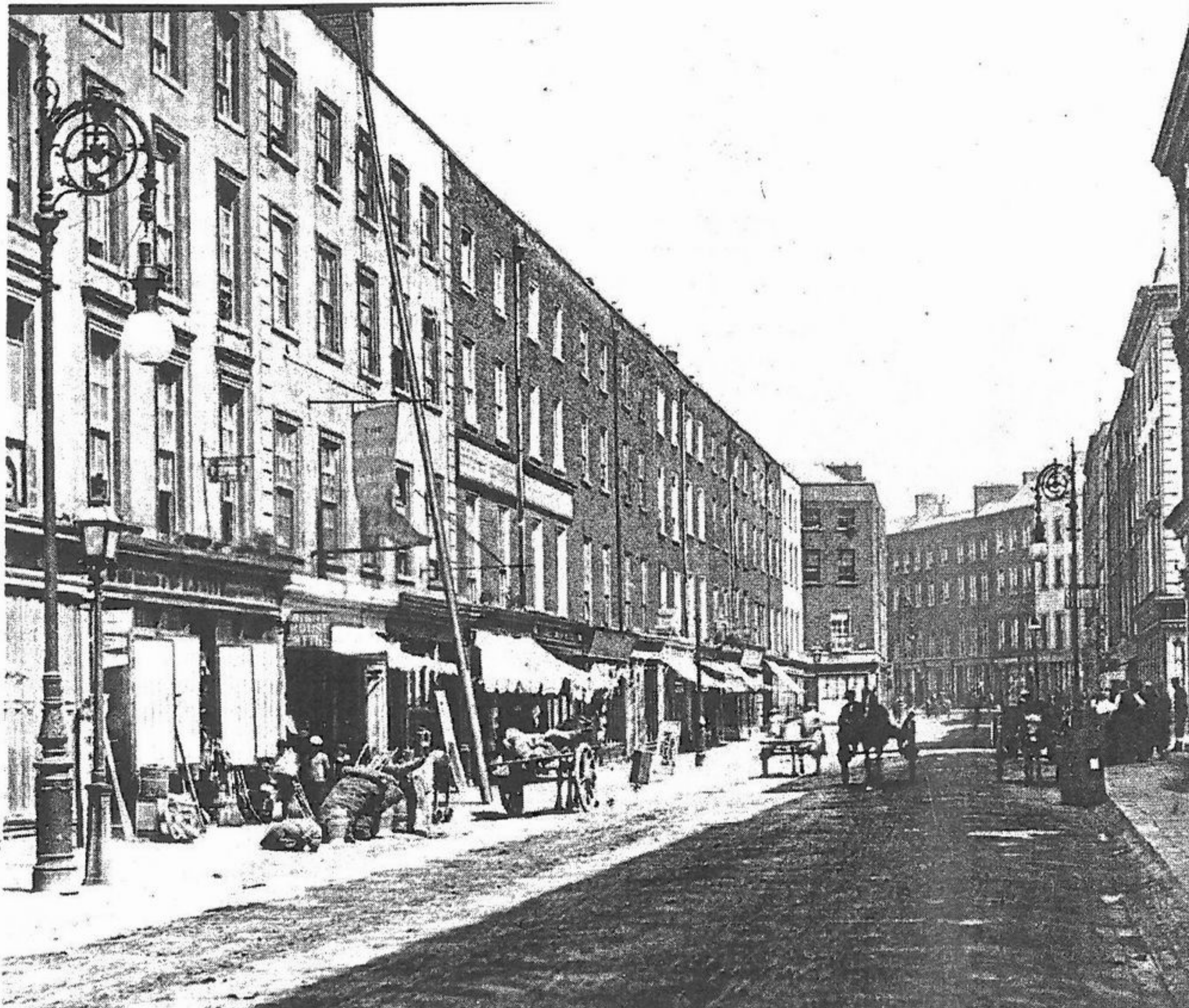
Patrick and Rutland Streets in Limerick city. Road surfaces in 1916 were soft limestone chip which turned to mud of dust, depending on the weather conditions of the day. On wetter days, they were described as 'rivers of slimy mud' PICTURE COURTESY OF LIMERICK ARCHIVES
