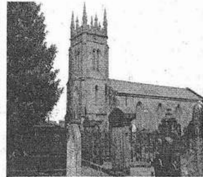
St Munchin's belfry, pinnacles and tower were all restored by the Civic Trust
