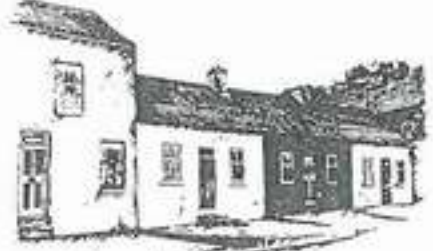
Verdant Place Reclamation of site around Medieval City Wall
