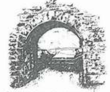
Medieval city walls at Johnsgate Restoration work
