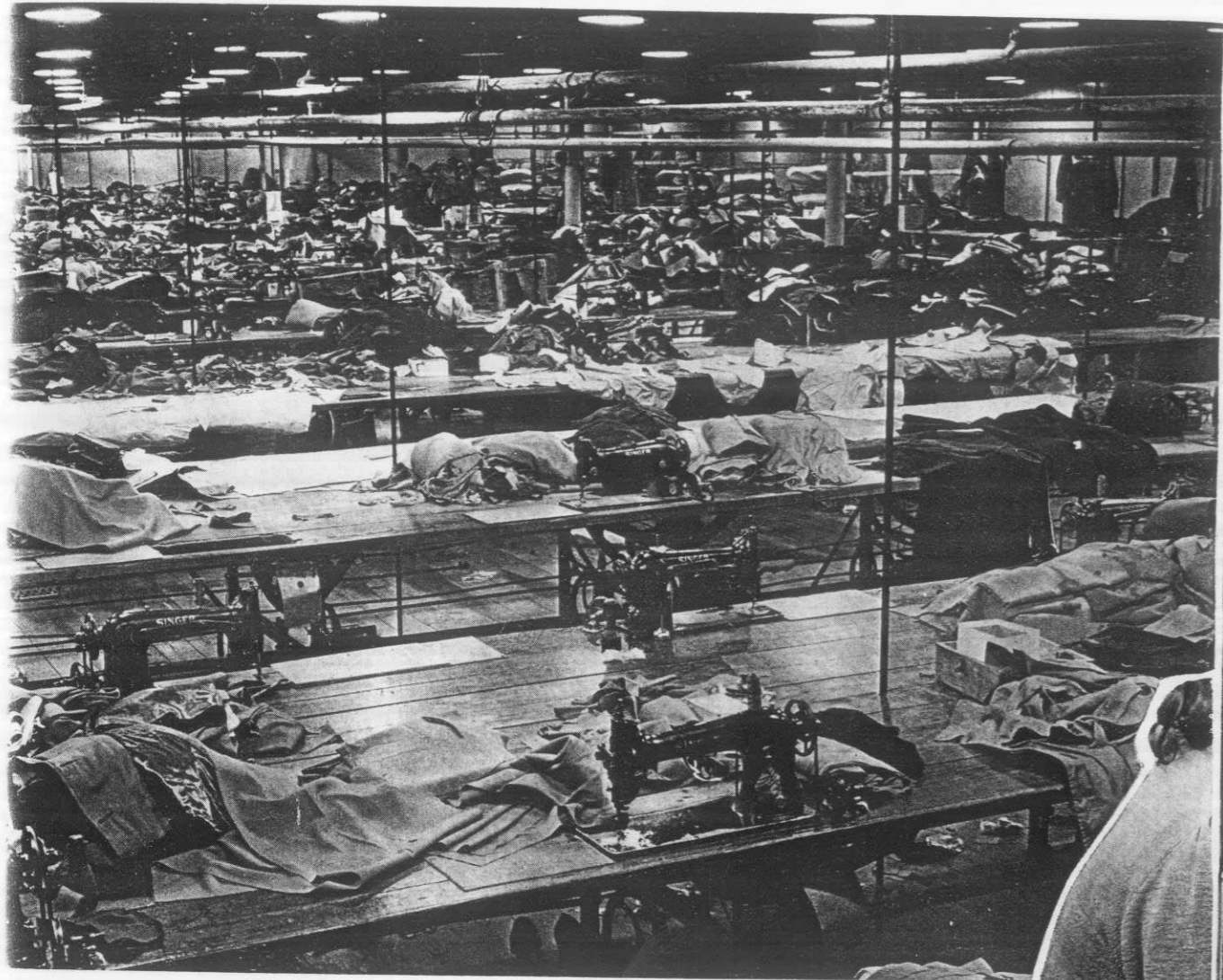
The general machine room photographed at night
