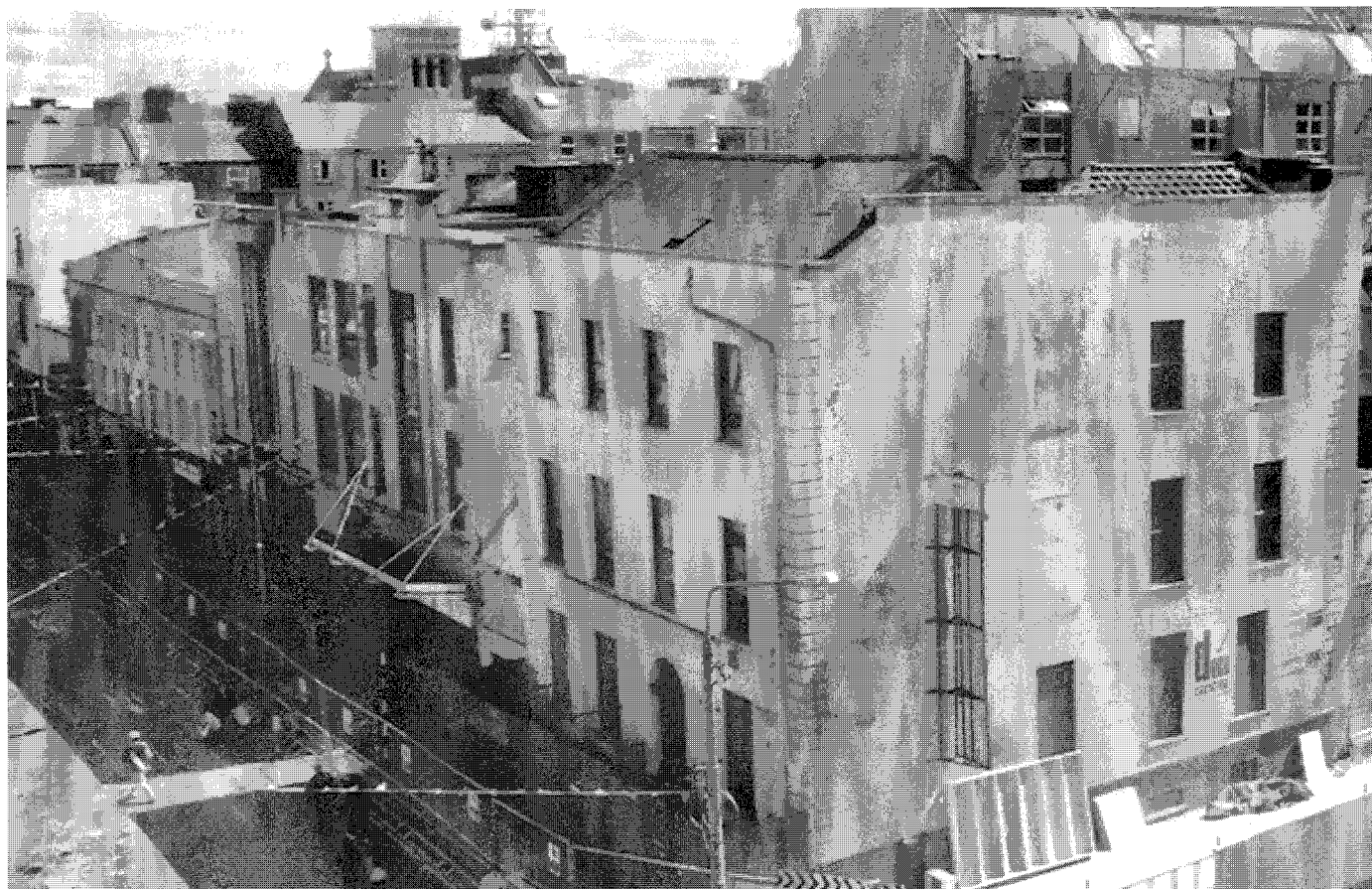
View of hospital building before demolition, 2006
