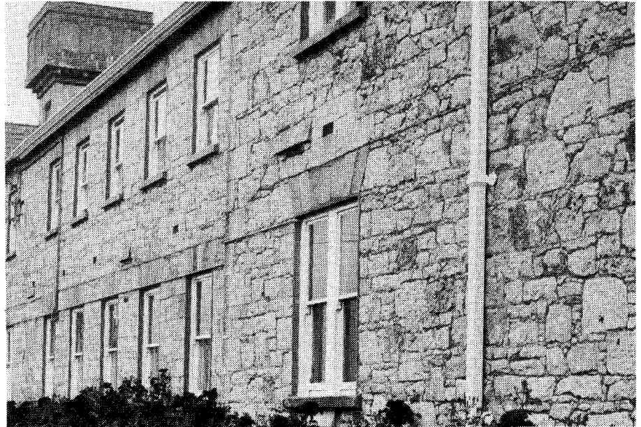
Part of the front wall of the Newcastlewest Workhouse.
