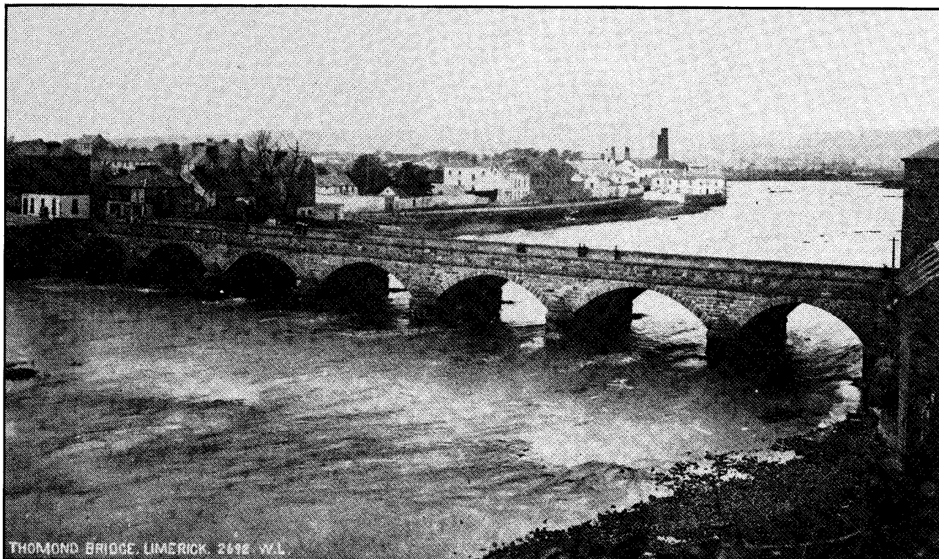
Thomond Bridge, with the distillery in the background.
