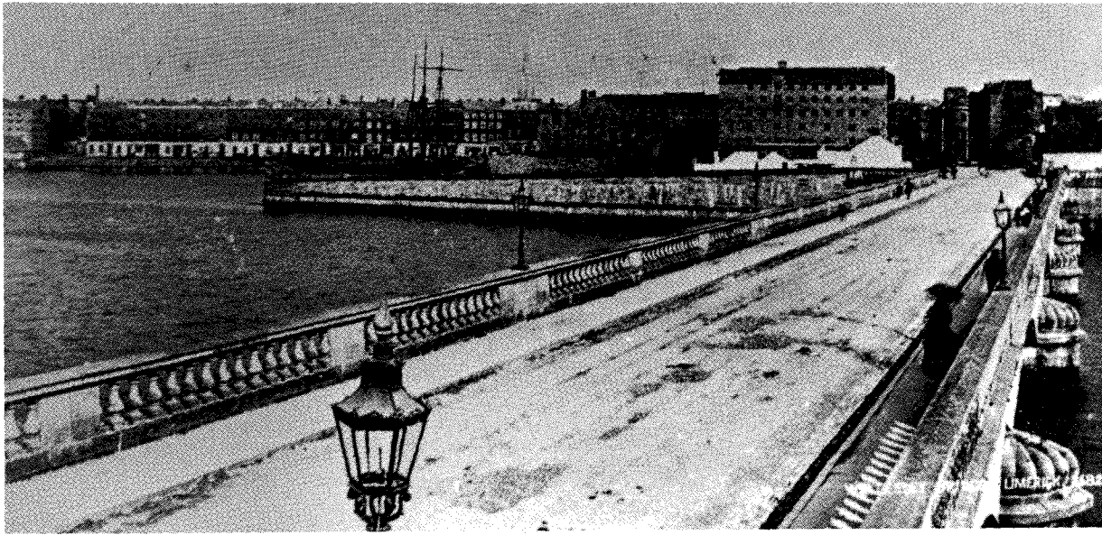
The Wellesley Bridge, with Arthur's Quay in the background.
