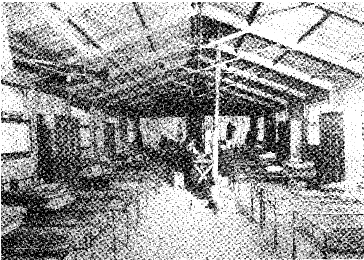
Some of the better sleeping quarters for Shannon Scheme workers.
