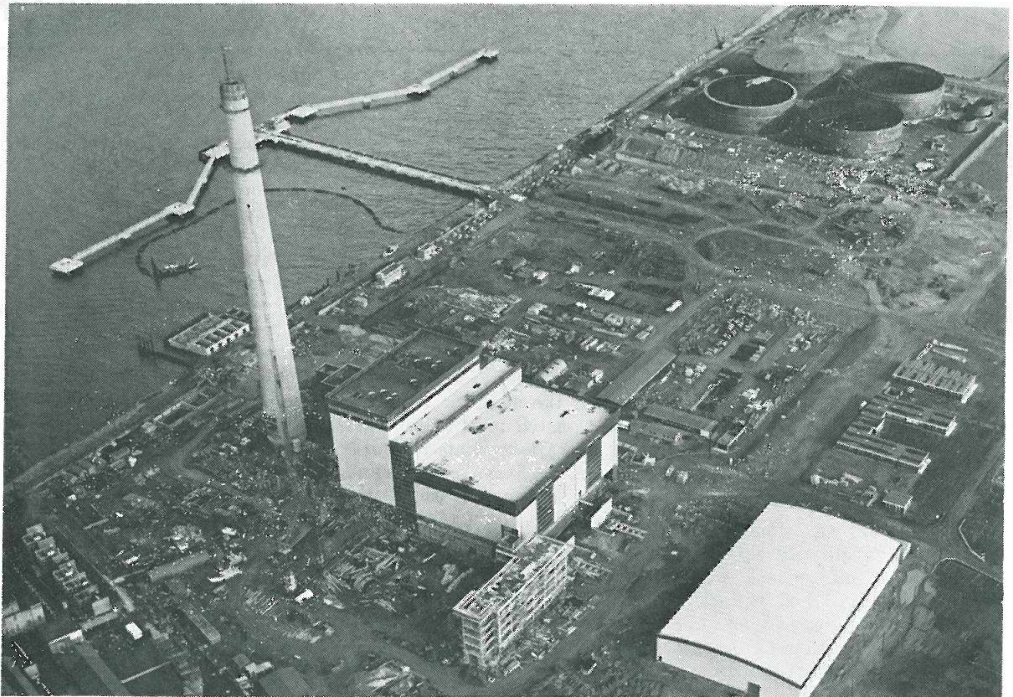
The E.S.B. Pigeon House 'B' generating station now under construction at Ringsend in Dublin.
