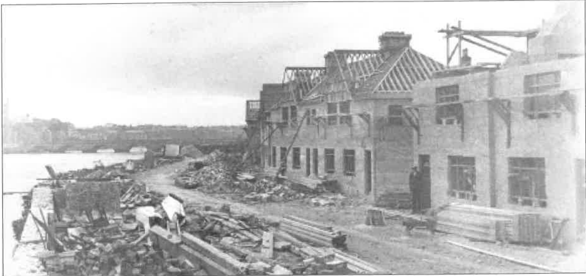
New houses being constructed on the old distillery site in Thomondgate. (Courtesy of Limerick Museum).
